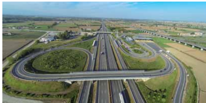
Improvement work and upgrades A4 Turin - Novara Est section (45 km)
