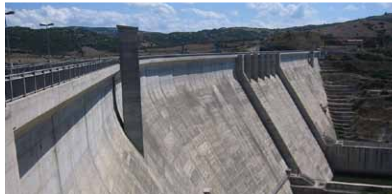
Dam on Tirso river (Oristano)
